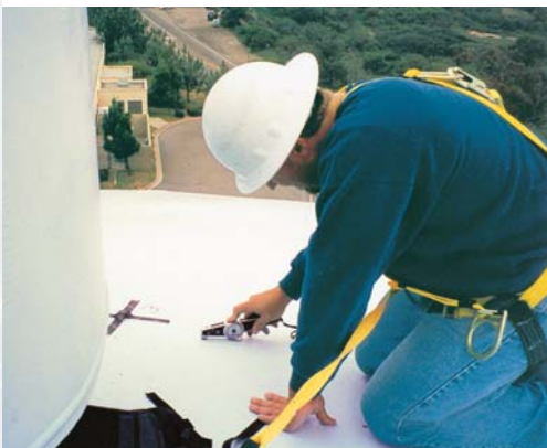
Above: Tank Inspection Right: Advanced Rectifier Design
